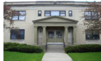
Hospitality House, 271 Central Ave., Albany
